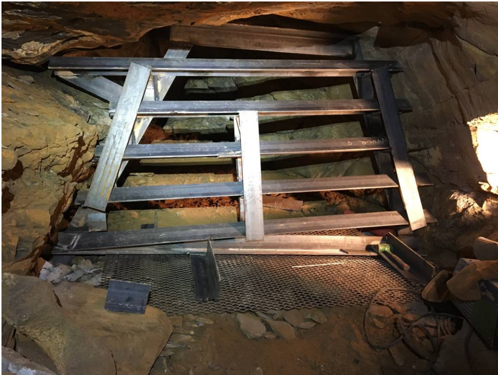
Figure 6. Completed bat-friendly gate at Ruth Cave.
